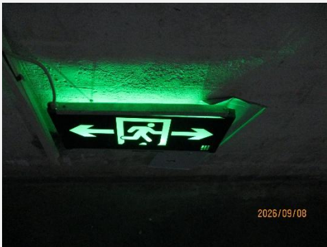
4-4: Exit route with marking
